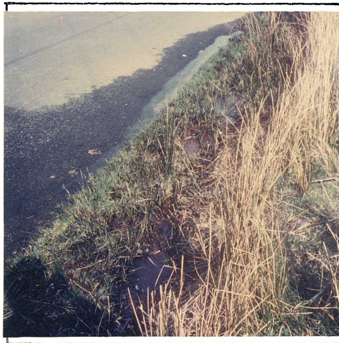
Plate 3:24 Sychnant Pass : following heavy rainfall water overflowed onto the road and thin layers of ochre developed on the road surface. On drying these left a red stain.
