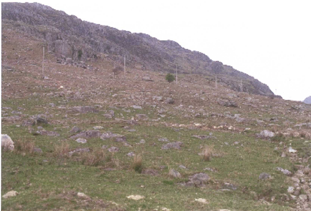
Figure 2.2: Power line in an Upland Area.
