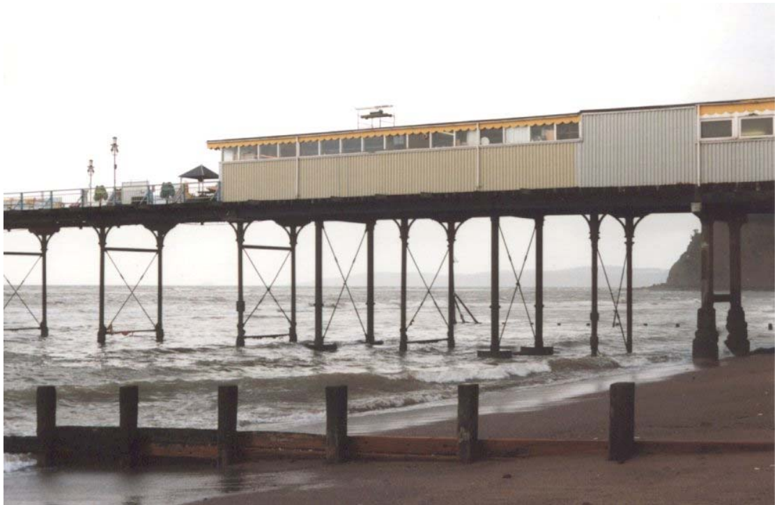
Figure 3.5.1 The X-Band radar mounted on the roof of Teignmouth Pier during the 1999 COAST3D experiment.
