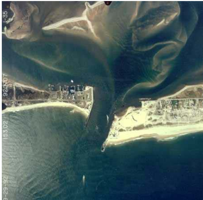
Figure 8.3.5 A photograph of Shinnecock Inlet in the USA in which the erosion of the beach downdrift (left) of the inlet is clear.
