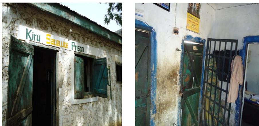
Picture 5.13: Physical structures of KSP
