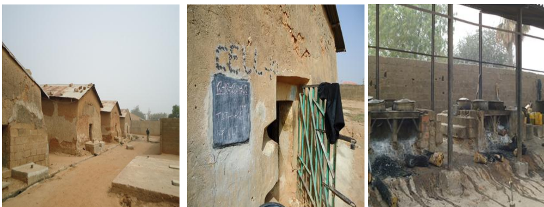
Picture: 5.3: Structures of large-size dorms, and a kitchen at KCP.
