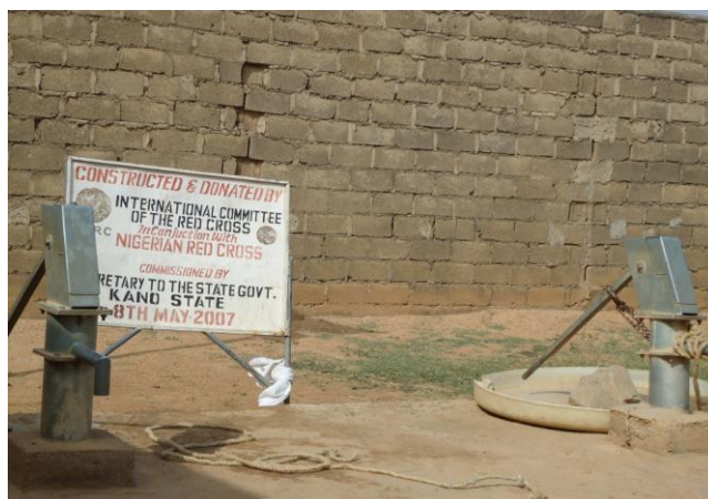
Picture 7.1: A hand-pump water supply constructed by ICRC
