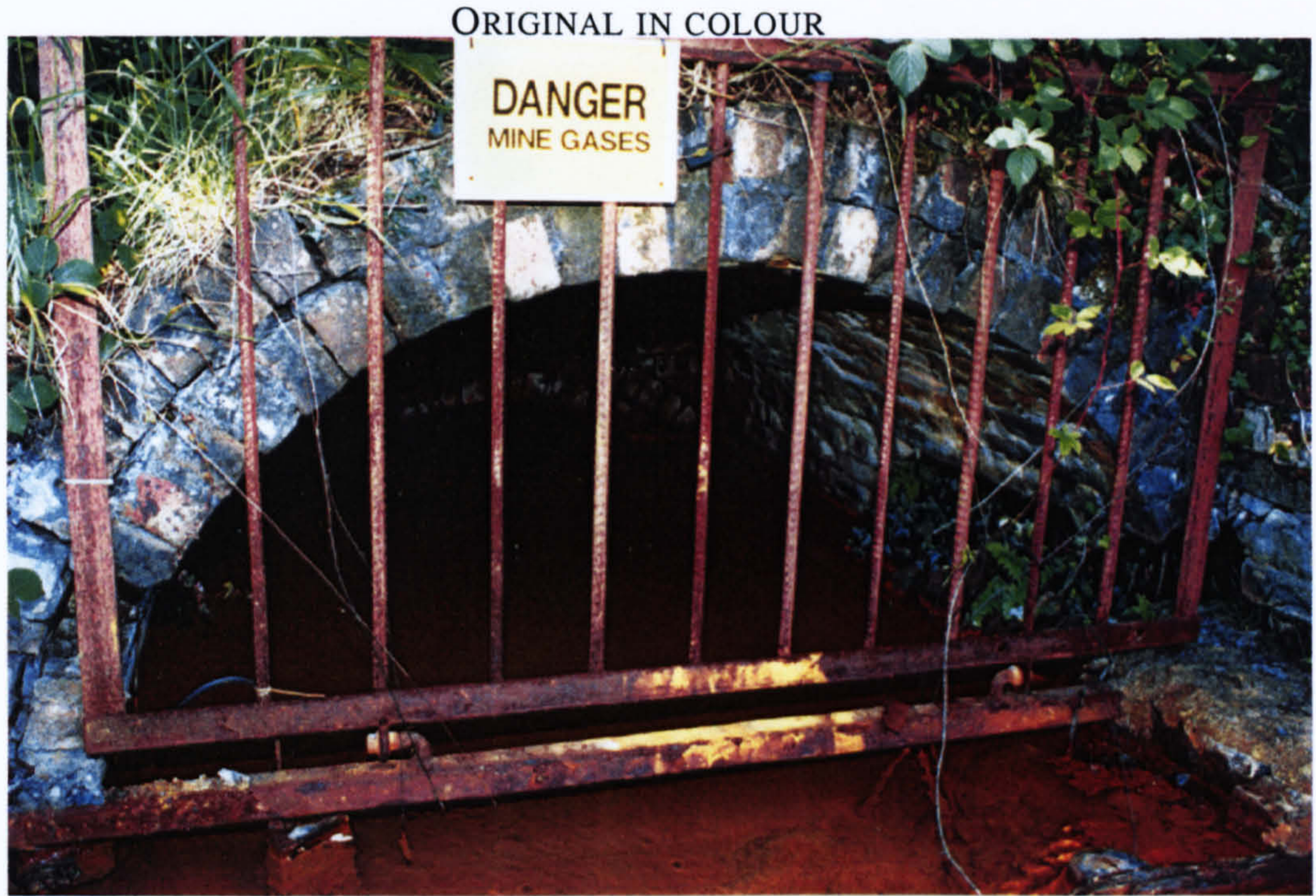
Figure 2.2: Ynysarwed mine water discharge adit.
