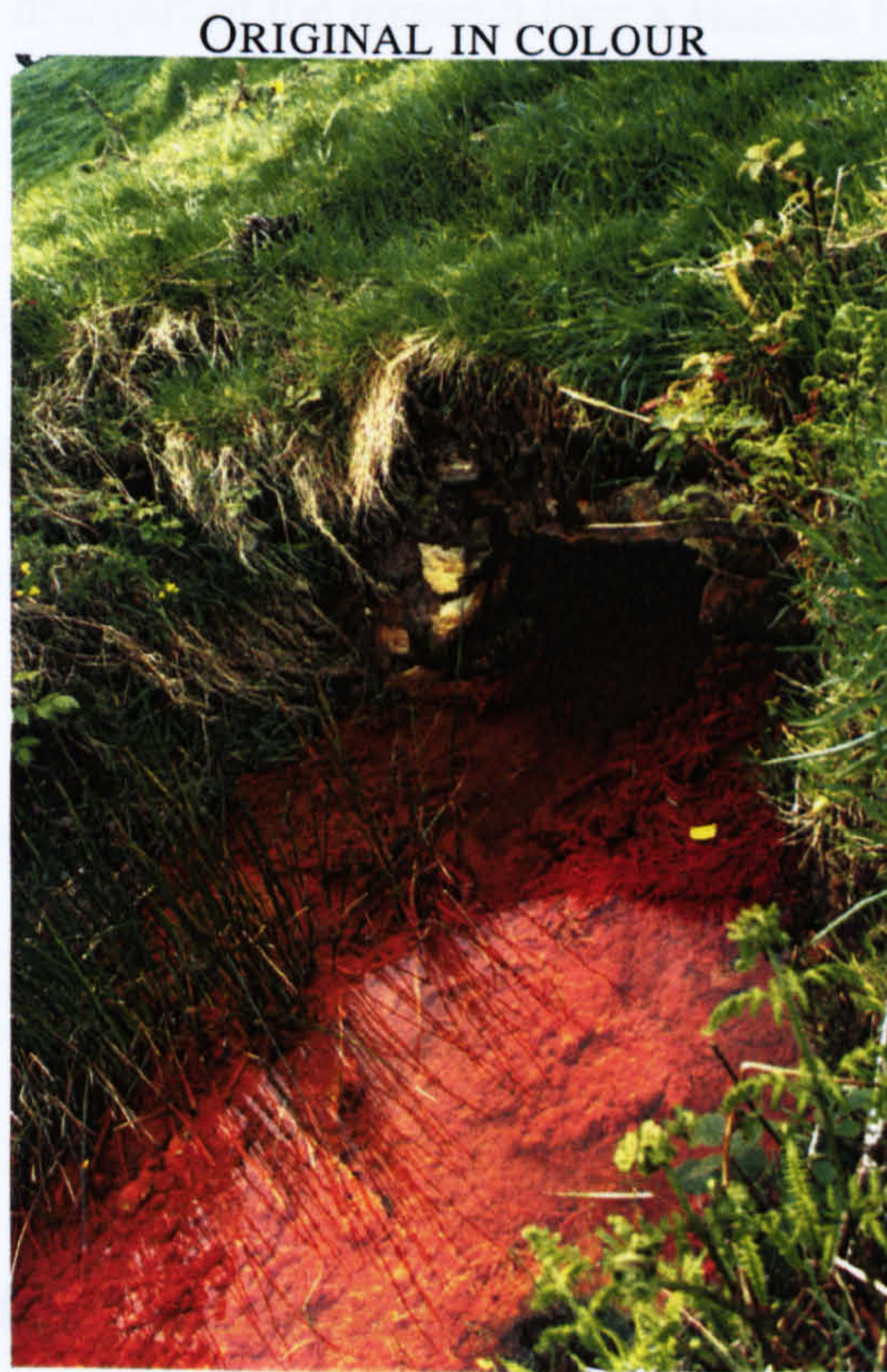
Figure 2.6: Dyffryn Adda mine drainage discharge point.
