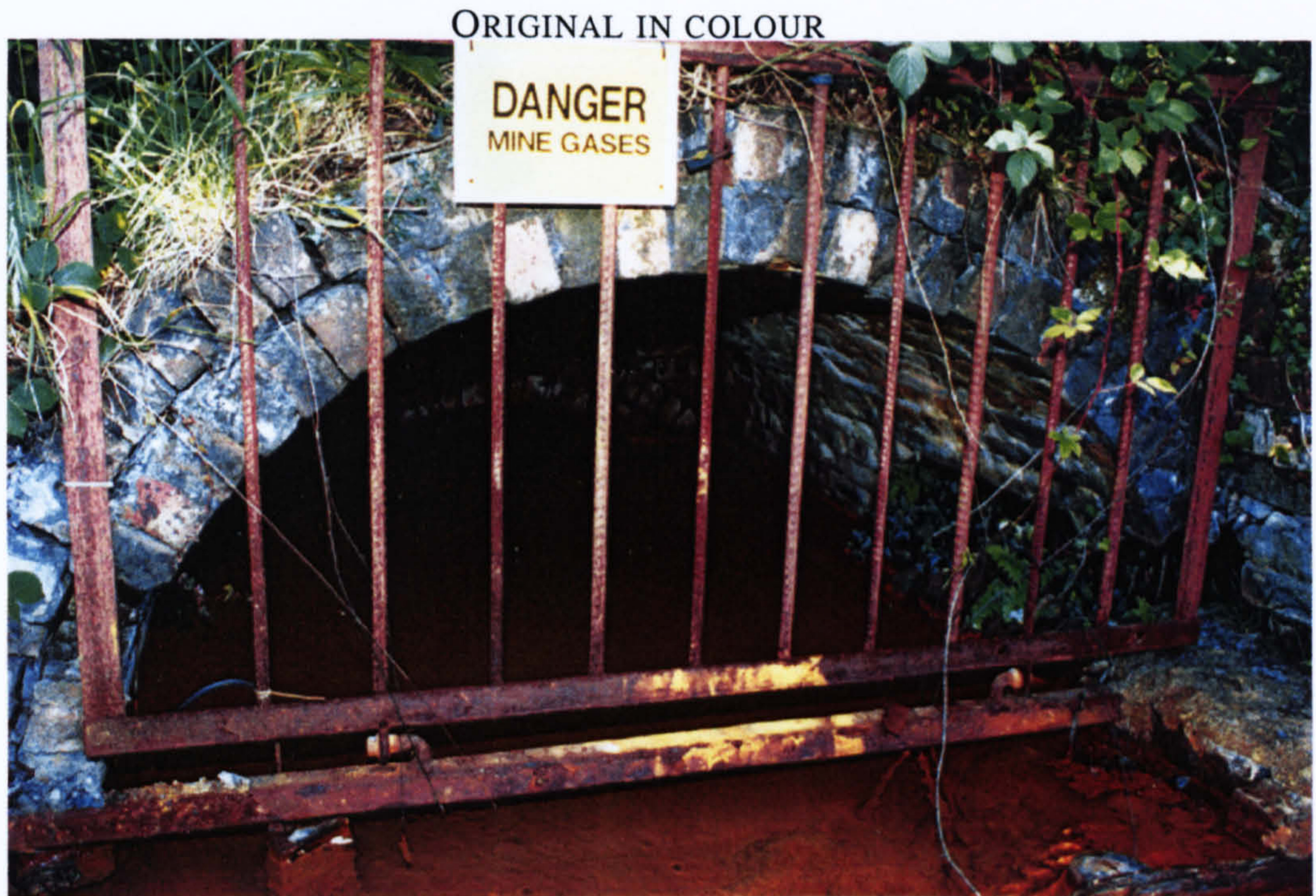
Figure 2.2: Ynysarwed mine water discharge adit.
