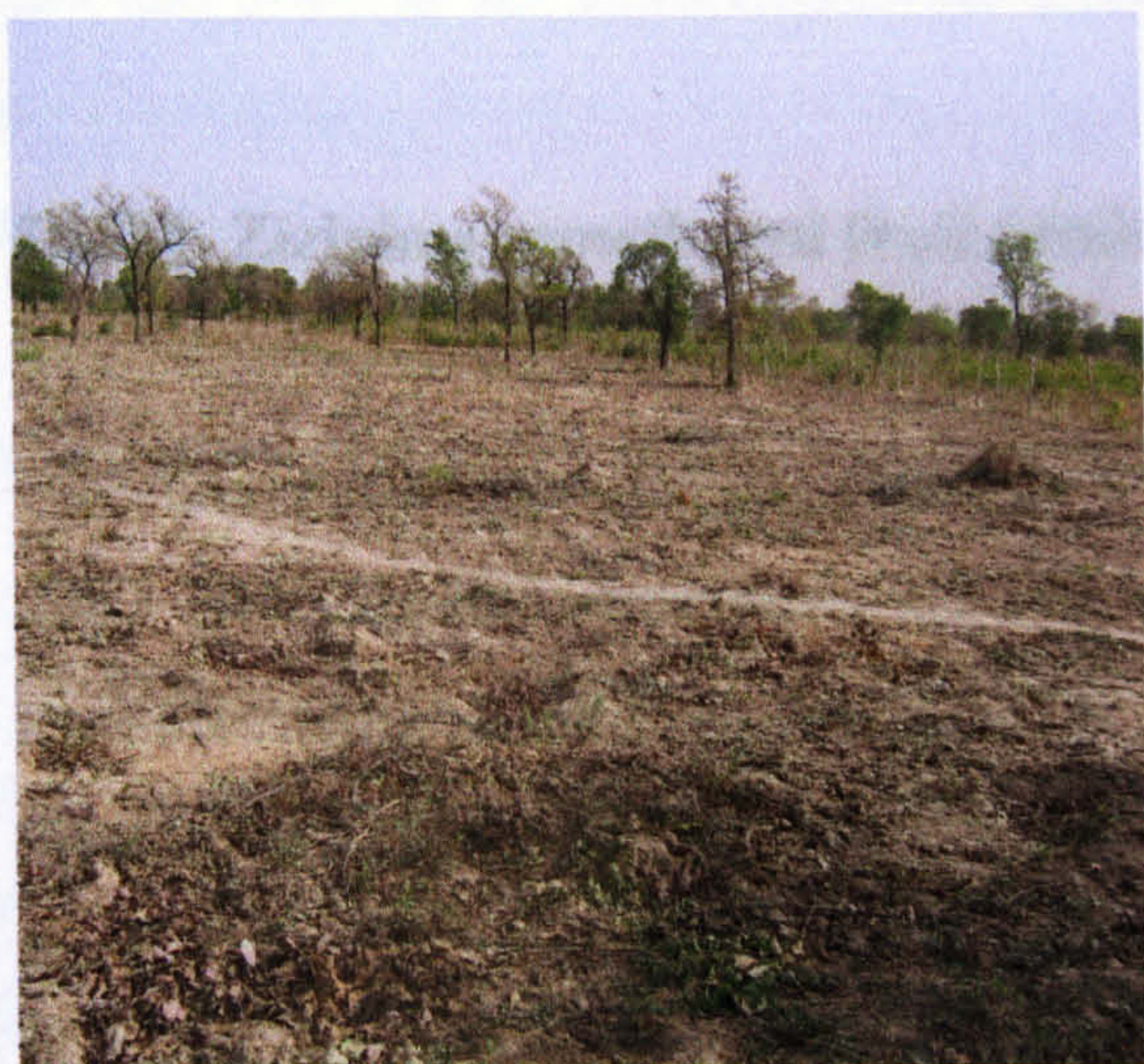
a) Site prepared for plantation
