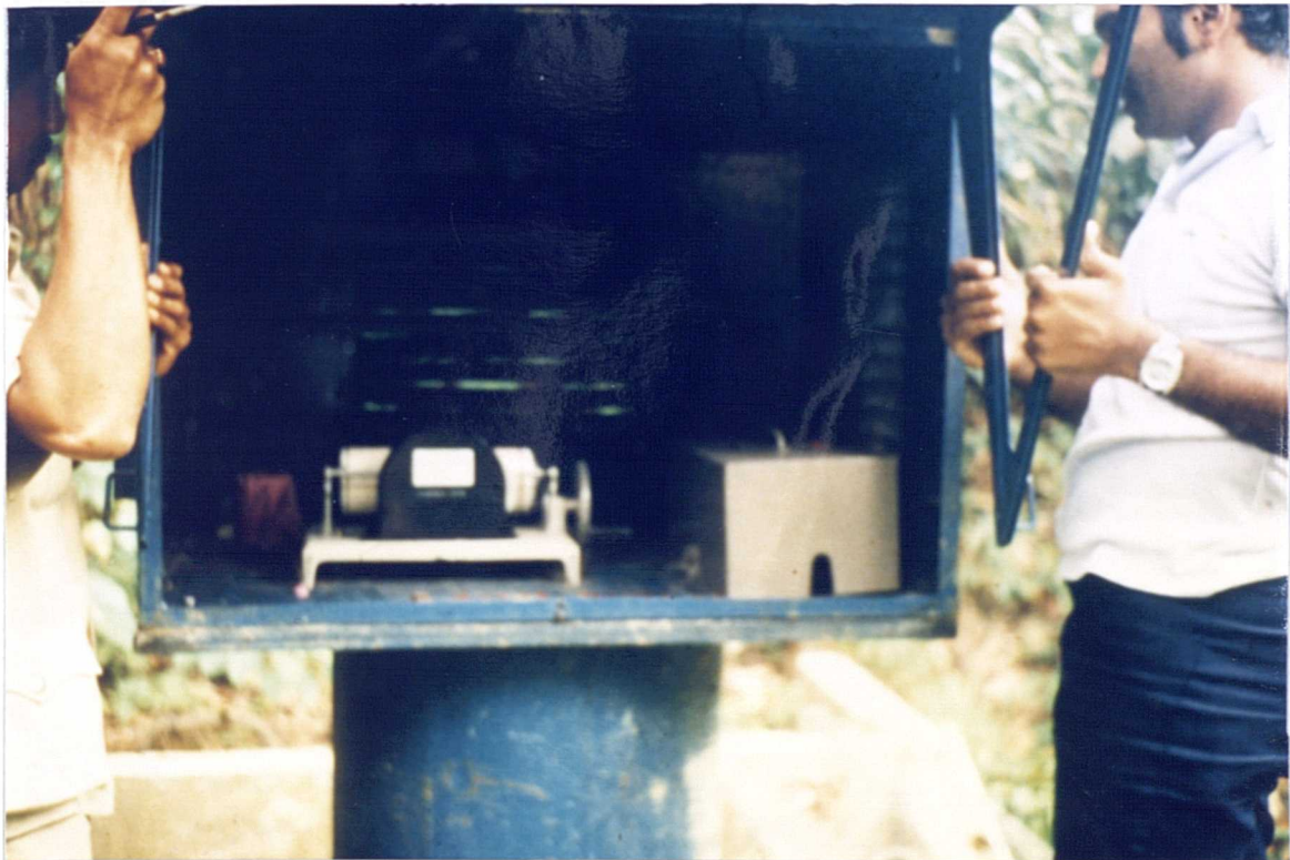
Plate 4.4 Stilling well and water level recorder at weir basin
