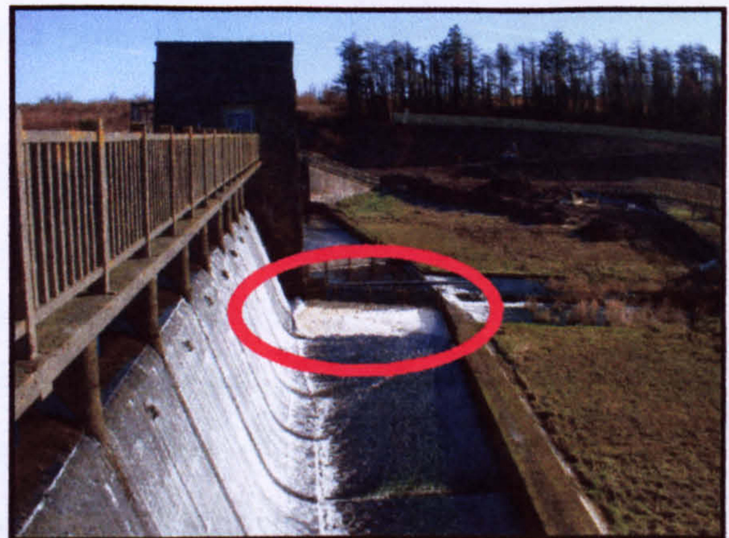
Figure 2.02 – Cefni lake dam and outflow
