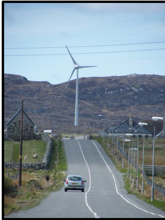
Figure 4.2 Picture showing the Cuibhle an Fhortain (The Wheel of Fortune) turbine from north Siabost
