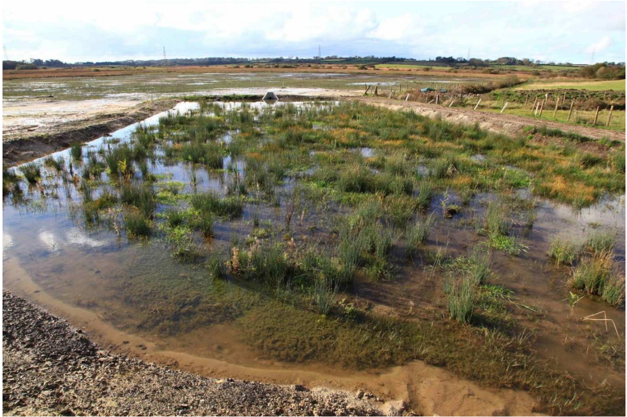
Figure 4.7 – Completed system at Cae Gwyn.
