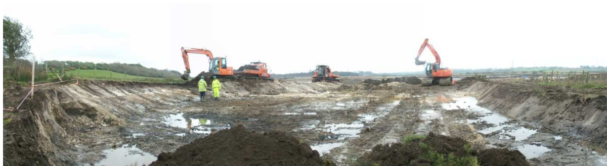
Figure 4.6 – View from the inlet zone during construction phase with civil engineering contractors at Cae Gwyn FWS CW.
