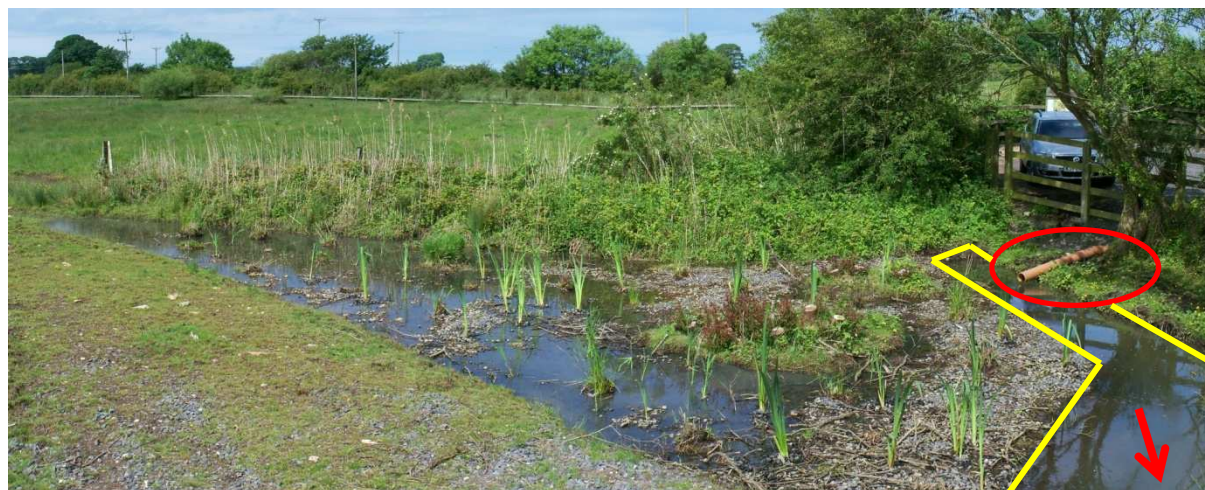
Figure 4.4 - Bodeilio HSSF system NitraBAR hybrid planted with Iris pseudacorus .
