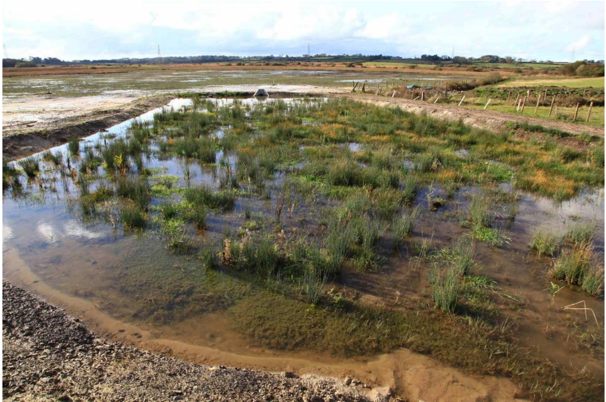
Figure 4.7 – Completed system at Cae Gwyn.
