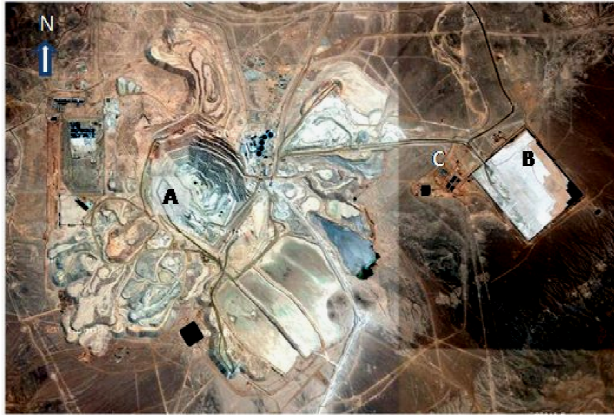
Figure 3.1. Satellite image of Escondida mine showing the location of relevant processes. Pit (A), Bioheaps (B) and solvent extraction facility (C).
