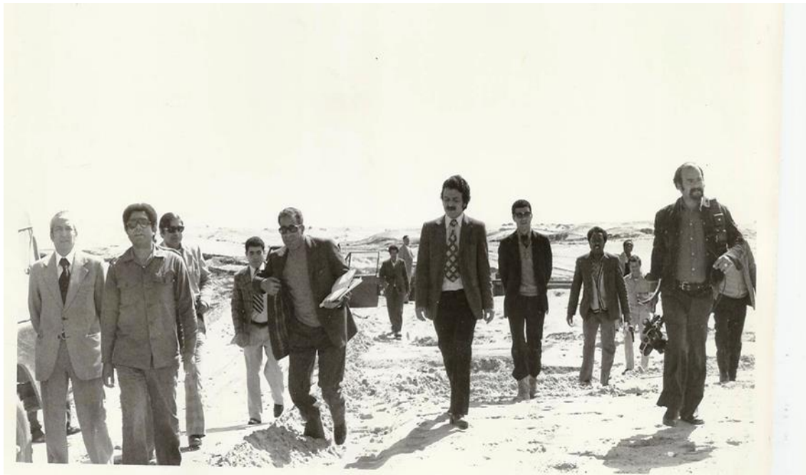
Figure 2.22: Government officials supervise the process of sand dunes stabilization (02/02/ 1972).
