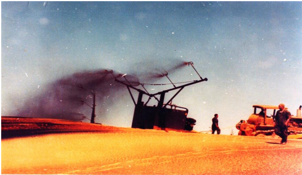
Figure 2.18: Sand dunes stabilization by using crude oil: The process of sand dunes stabilization by bitumen spray by a bulldozer which pulled the tank over the dunes ,in Al Atayah village in Algarabulli district in 1971 (Khatabi, 1981).
