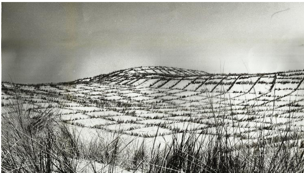
Figure 2.16: Sand dunes stabilization by dry plant materials in second stage: Illustration of sand dune after stabilized dry plant materials in Al Atayah village in Algarabulli district by Imperata cylindrica and Aristida pungens 1968 (Ajaj, 1982).
