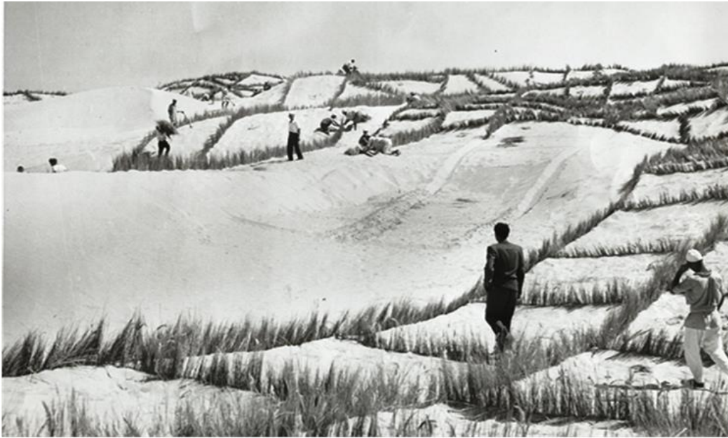
Figure 2.15: Sand dunes stabilization using dry plant materials first: Illustration of the process of sand dunes stabilization using Imperata cylindrica and Aristida pungens , Al- Atayah village in Algarabulli district in 1966 (Ajaj, 1982).
