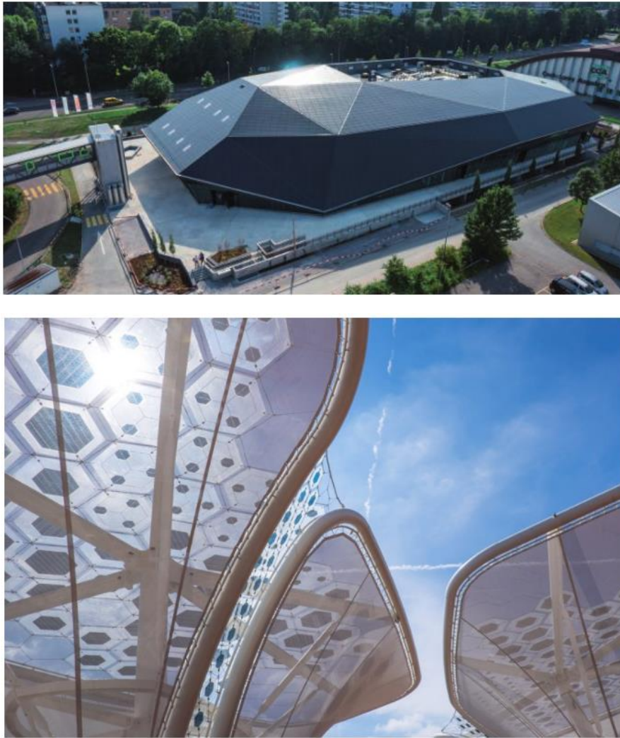
Figure 2.27 – Umweltarena Spreitenbach, 750 kWp BIPV envelope consisting of c-Si panels with an anti-reflective coating [28] (Top) and tree shape structure with transparent hexagonal OPV solar modules demonstrated during expo Milano 2015 [150] (Bottom).
