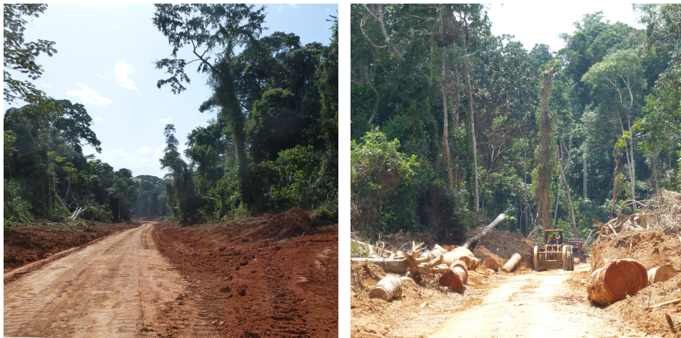
Figure 1.4 – Newly constructed logging roads in south east Cameroon and northern Republic of Congo. Left: Primary road, providing permanent access to the forest. Right: secondary (dead-end) road built for temporary use to collect timber from log landings (here stored on the road side).
