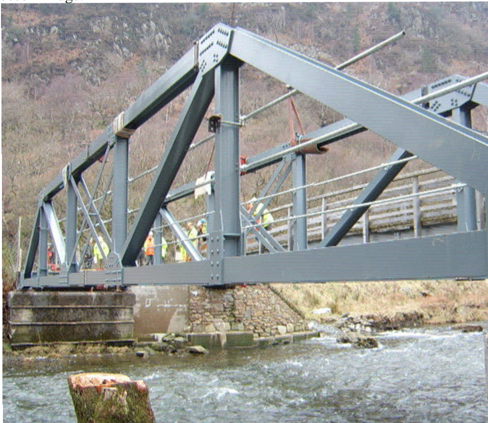
6.9. Bryn y Felin Bridge constructed and installed by the Brunswick Ironworks. Reproduced from the Brunswick archives with their kind permission 2011.
