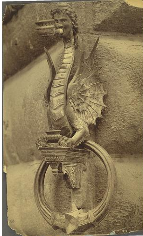
Image 3.1. Wrought iron torch holder/horse tether created by Niccolo Grosso circa 1490 for the Strozzi Place, Florence. Image reproduced from the Free Cornell University Library USA ( http://www.flickr.com/photos/cornelluniversitylibrary/361113161 )
