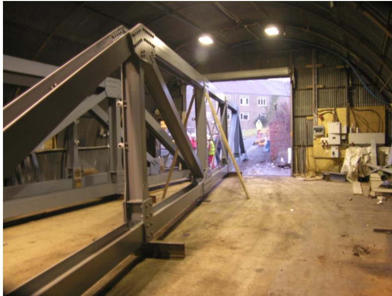
Photo 3.55. Under construction Brunswick Ironworks 2008 the Pont Croesor Bridge. Reproduced from the Brunswick Archive with their permission.
