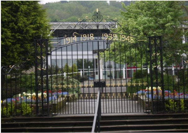
Photo 3.20. Gates Holywell Flintshire made by DJ Williams on the left complete with lanterns circa 1946 and on the right the gates restored by Flintshire County Council 2006. Photographed by Pam Smith 2007.
