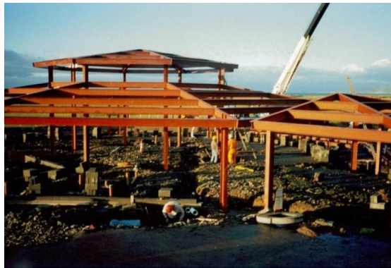
Photo 3.52. Structural steel work for Llyn y Gele Clubhouse. Reproduced by kind permission of the Williams family.
