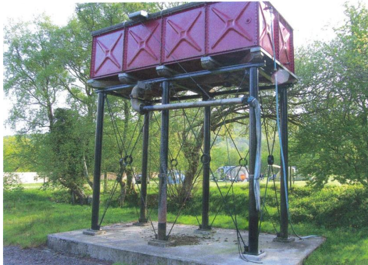
7.1.4. Waunfawr Water Tower.
