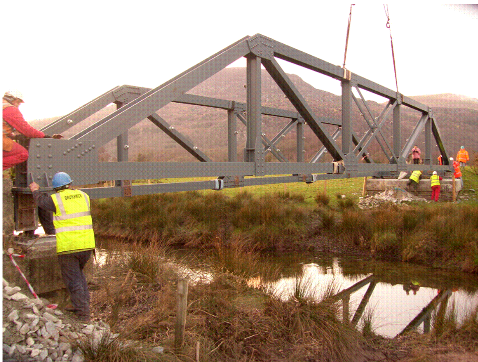
Photo 3.56. Installation of Dylif Bridge March 2007. From the Brunswick Ironworks Archive reproduced with their kind permission.
