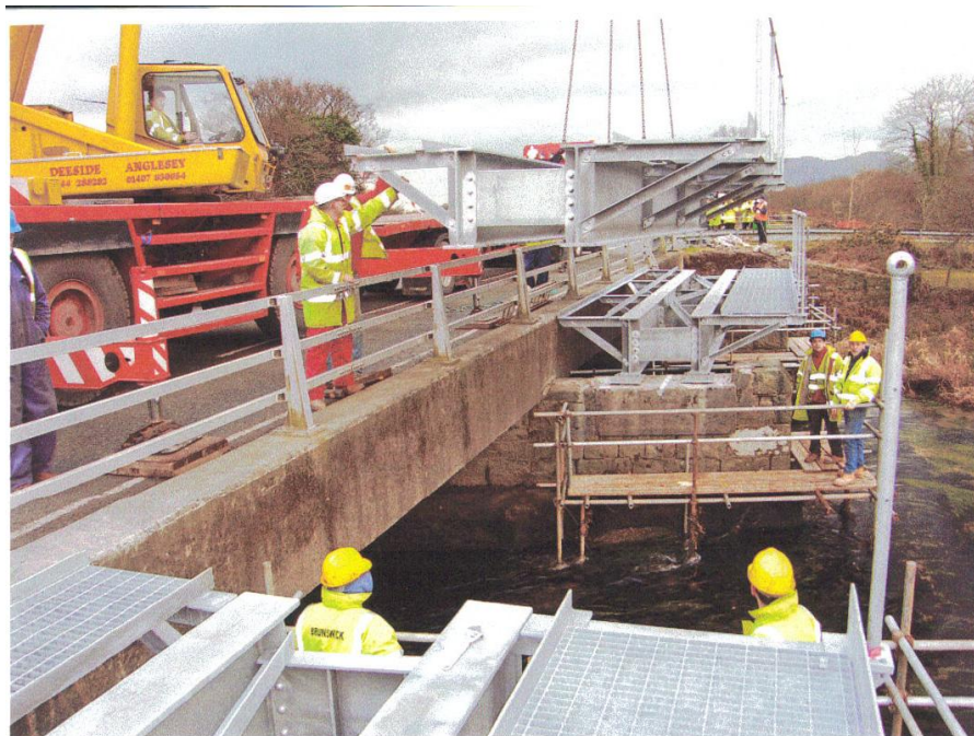
Photo 3.54. Nantmor Bridge installation October 2006. Reproduced from the Brunswick Ironworks archive reproduced with their kind permission.
