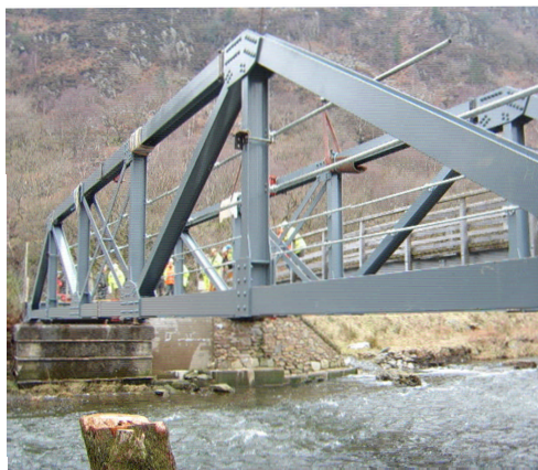
Photo 5.12. Bryn y Felin Bridge installation Brunswick Ironworks. Photograph from the Brunswick archive reproduced with their kind permission.
