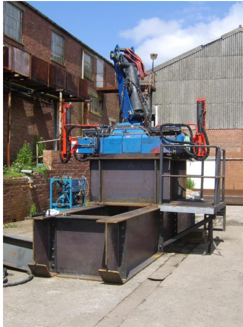
7.2. Steel frame fabricated to support telescopic jib.
