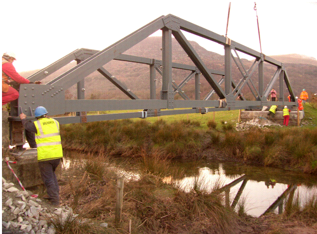
7.0. One of five bridges fabricated, transported and erected. Client-Welsh Highland Railway.
