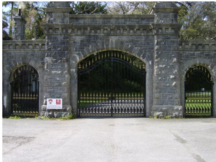
Photo 3.16. Vaynol Estate Gates Bangor Gwynedd. Photographed by Pam Smith 2008
