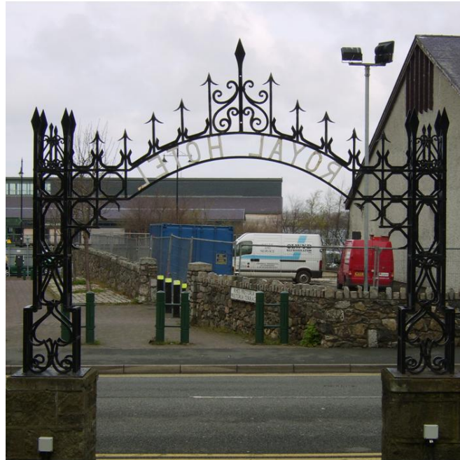
3.14. The gates at the Celtic Royal Hotel created circa 1930 and restored by the company in 2009. Photographed by Pam Smith 2009
