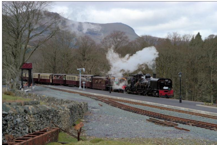
Photo 3. 58. Beddgelert Station showing the water crane and water tower fabricated by Brunswick Ironworks for the Welsh Highland Railway. Photograph by Peter Johnson (2009) reproduced with his kind permission.
