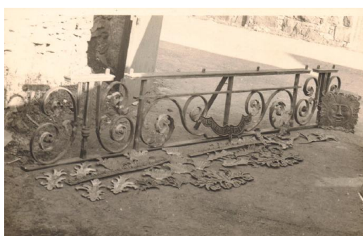
3.35. Original photograph of part of the gates dismantled and awaiting repair at the Brunswick Ironworks, reproduced from the Williams family archive with their kind permission.
