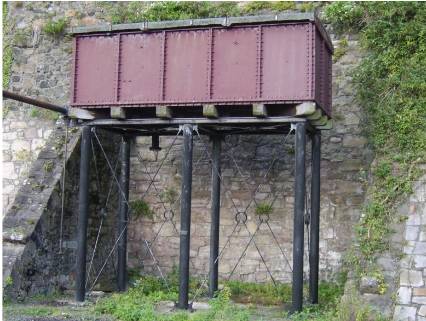
6.8. Water Tank built by Brunswick Ironworks at Caernarfon Station for the Welsh Highland Railway. Photographed by Pam Smith.
