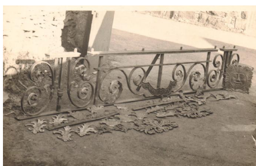
3.35. Original photograph of part of the gates dismantled and awaiting repair at the Brunswick Ironworks, reproduced from the Williams family archive with their kind permission.
