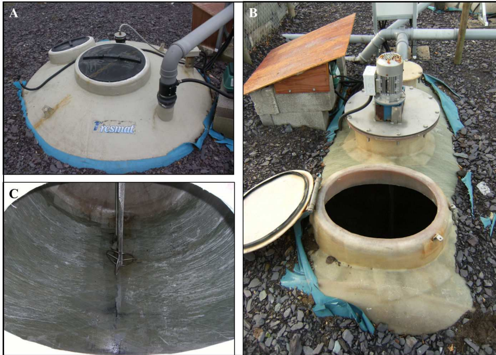
Figure 2: Photographs of the old, or vertical, (A) and new, or horizontal, (B) bio-reduction vessels and the inside of one of the horizontal bio-reduction vessels showing the agitator, or mixing paddle (C).
