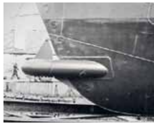
▲ Clockwise from top left: launching the first Prince Madog's hull at the Ramsey yard before the backward-sloping stern was altered; the vessel at Port Dinorwic (Felinheli) dry dock in her original black livery; the bow echo sounder transducer fairing seen during the build. BANGOR UNIVERSITY & IVOR REES
