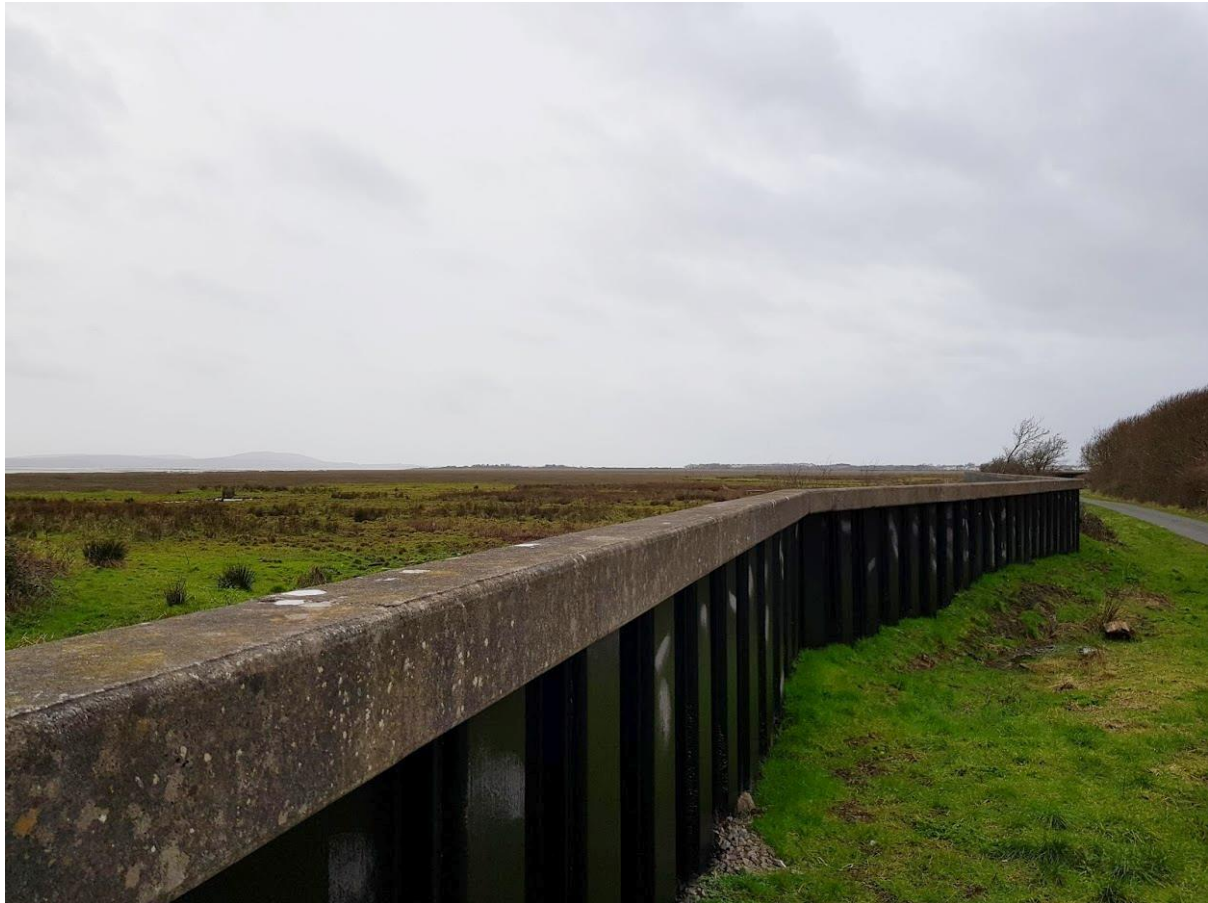
Supplementary Figure S7: Low-crested (approx.. 1m), narrow coastal defence walls such as this one between Loughor and Llanelli may be absent within the model domains due to their small size.
