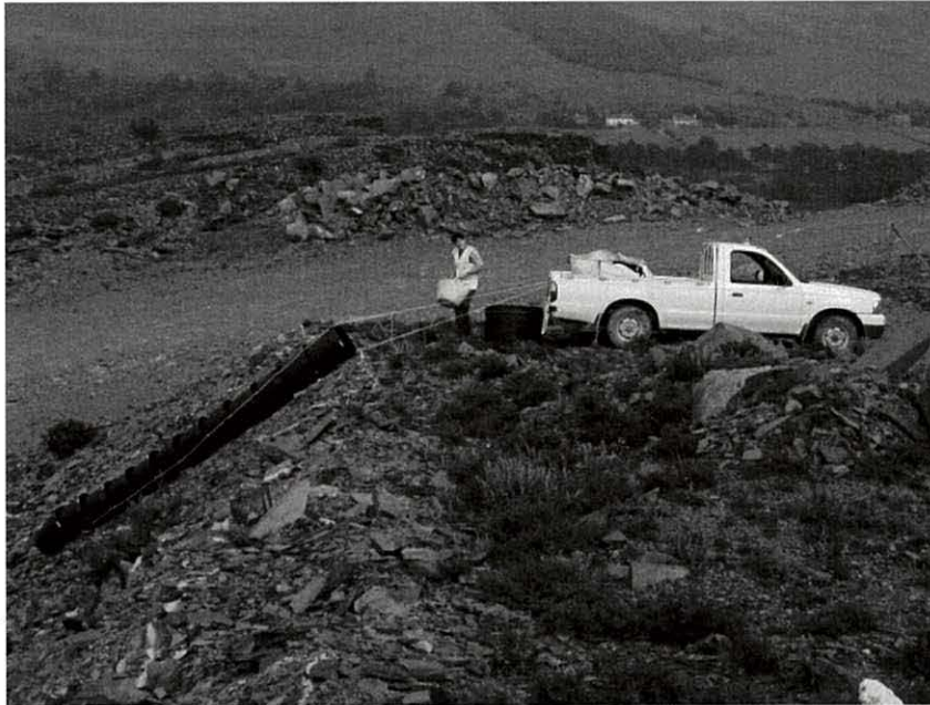
Plate 12 Material application chute connected to the pick-up tailgate
