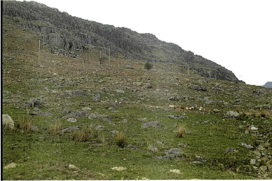
Figure 2.3: Power line in upland area
