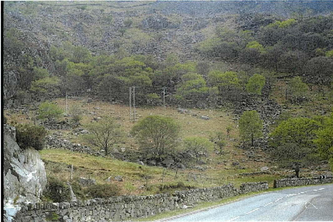
Figure 2.4: A difficult location for helicopter inspection due to the proximity of trees and a road
