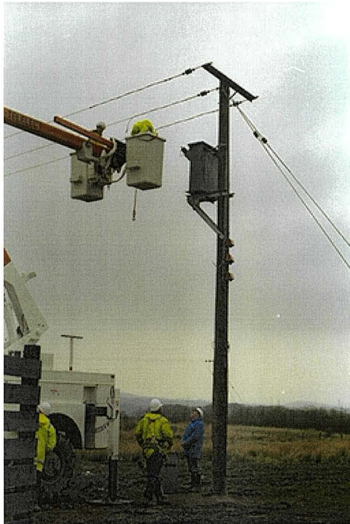
Figure 2.1: Line termination pole under repair
