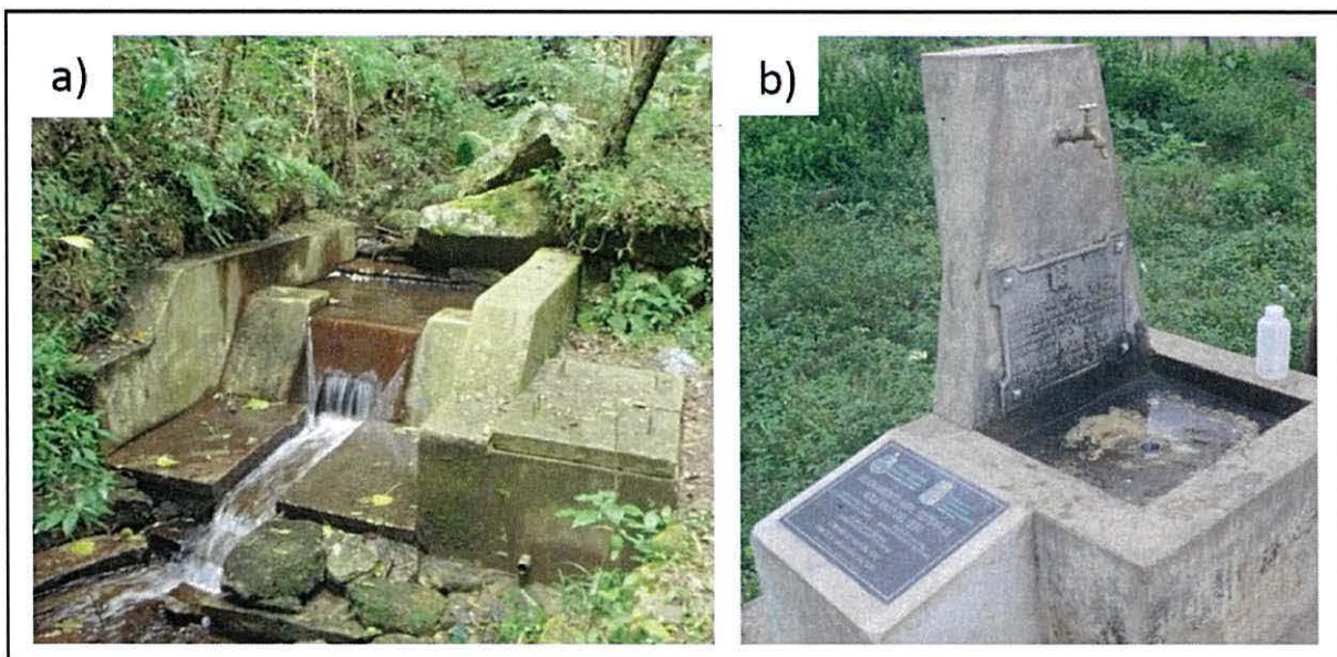
Figure 4.1. Examples of typical water supply systems in communities of the ANMI Río Grande. a) Water intake, Estancia Huaico (Vallegrande municipality); b) Community tap, central square, Vado del Yeso (Vallegrande municipality). Photographs: Edwin Pynegar.
