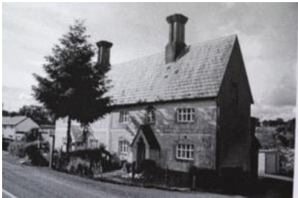
Nos 1 & 2, Concrete Cottages, Tregynon
