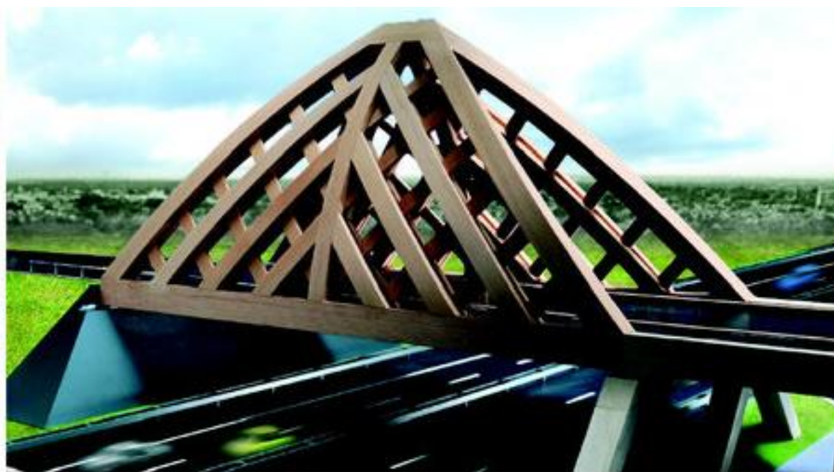
Figure 2-11 Highway bridge certified for 65 t load. Construction is made of acetylated glue laminated timber. Sneek, Netherlands. 319
