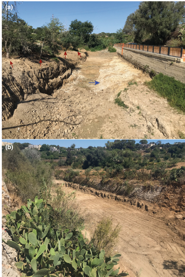
FIGURE 2 Pictures to demonstrate the constraints on efforts to ensure no refuges were left for crayfish during mechanical excavation. (a) Red arrows mark a handful of protected White Poplar Populus alba trees, which meant the bank could not be excavated (note the blue arrow shows where bedrock was struck during excavation). (b) Shows the traditional rubble wall alongside the valley system. A 0.5m buffer was left along such walls to retain their structural integrity. Crayfish could have survived in burrows alongside these buffers.
