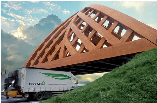
**Figure 4.** Glued laminated timber bridge, formed using acetylated radiata pine to carry traffic up to 65 t, built in 2008 at Sneek, the Netherlands (courtesy of Accsys Technologies plc)
