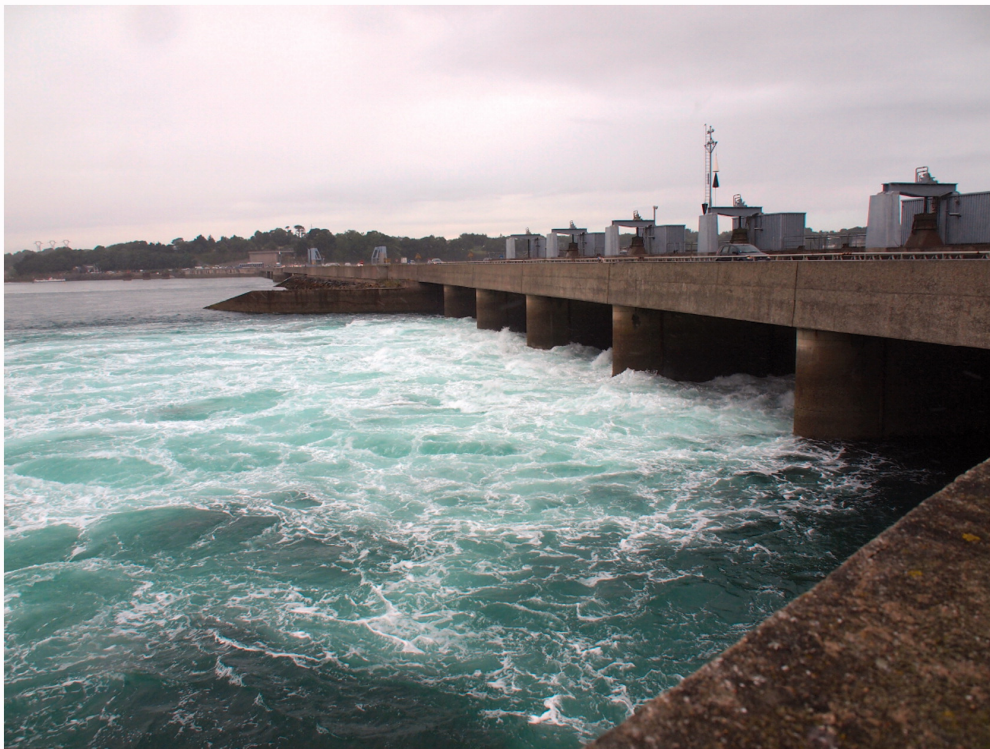
Figure 2.14: The La Rance barrage which is located on the French side of the English Channel.
