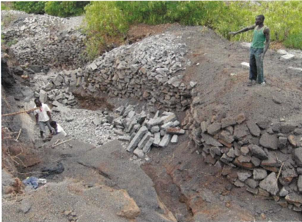
Plate 4. 4: Construction blocks mining in Holili, Tanzania
