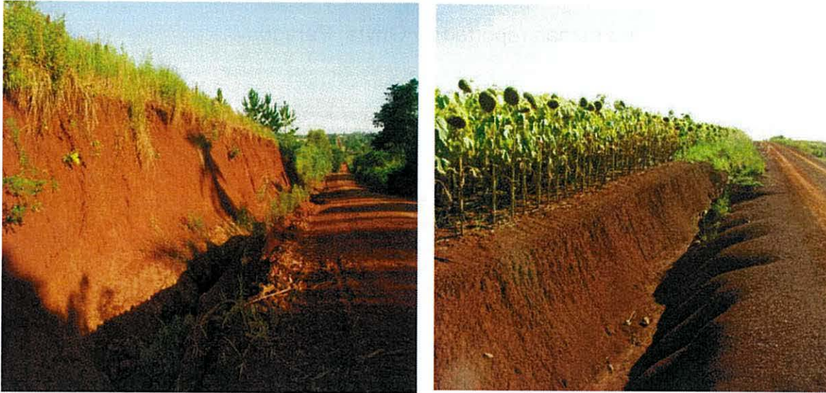
Figure 11. Photographs showing erosion in rural roads and cultivation areas. South 27°14,1 and West 55°46,9 / South 27°04 and West 55°53. (Mboi Cae) Itapua, Paraguay.
