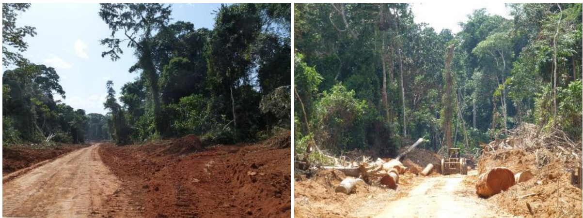
Figure 4. Newly constructed logging roads in south east Cameroon and northern Republic of Congo. Left: Primary road making permanent access to the forest. Right: secondary (dead-end) road built for temporary use to collect timber from log landings (here stored on the road side).
